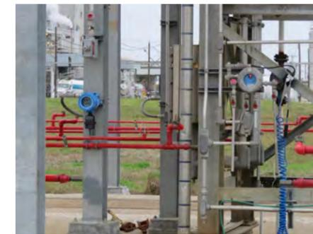
Figure 10. Fixed air monitoring (left) and bonding and grounding with continuity indicator (right) on a concrete loading/unloading pad. This pad is also equipped with fixed fire and vapor suppression.
