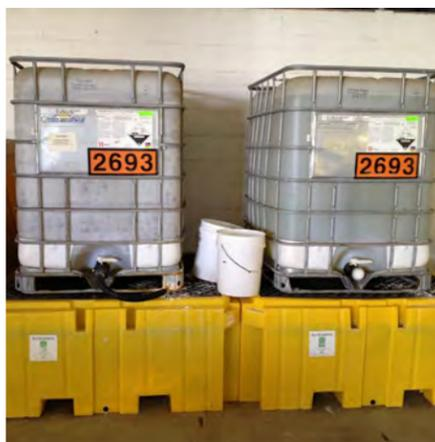
Figure 5. Composite or caged Intermediate Bulk Containers (IBCs) containing a corrosive material sitting on top of portable spill containment. Caged IBCs have a polyethylene plastic liner that is structurally supported by a tubular galvanized steel frame or cage.
